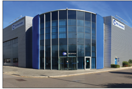
European Headquarters & Production Facility, Southampton, UK
